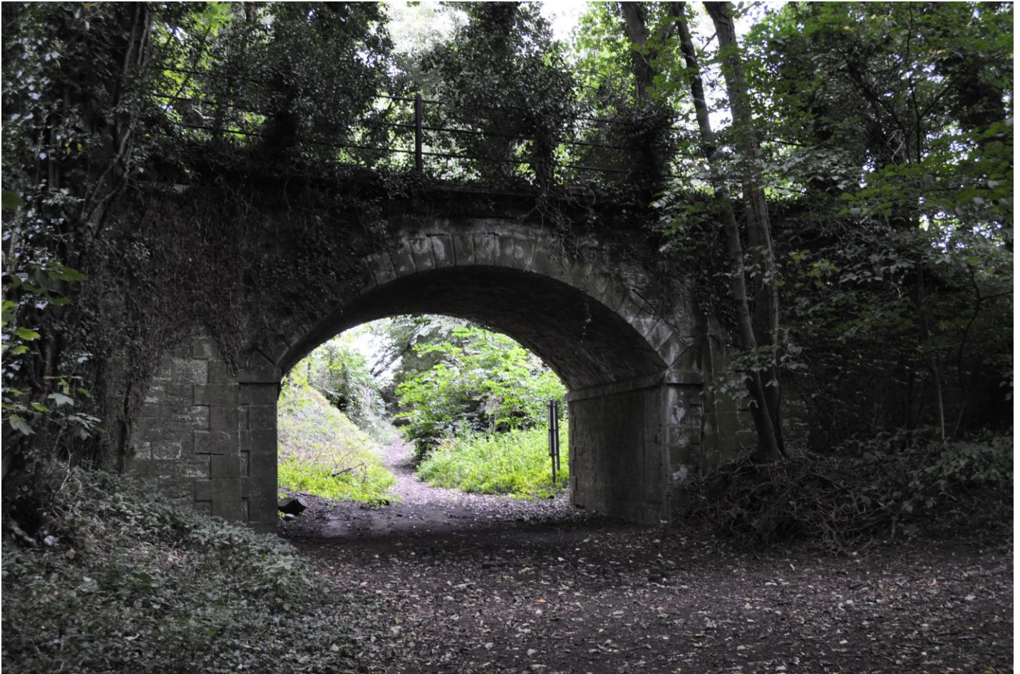
Figure 14: Skew Railway Arch at Watersmeet
